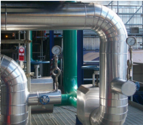
PIPING INSULATION
