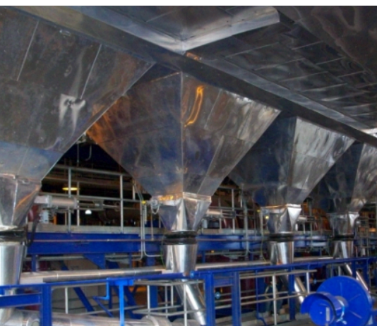
DUCTING INSULATION
